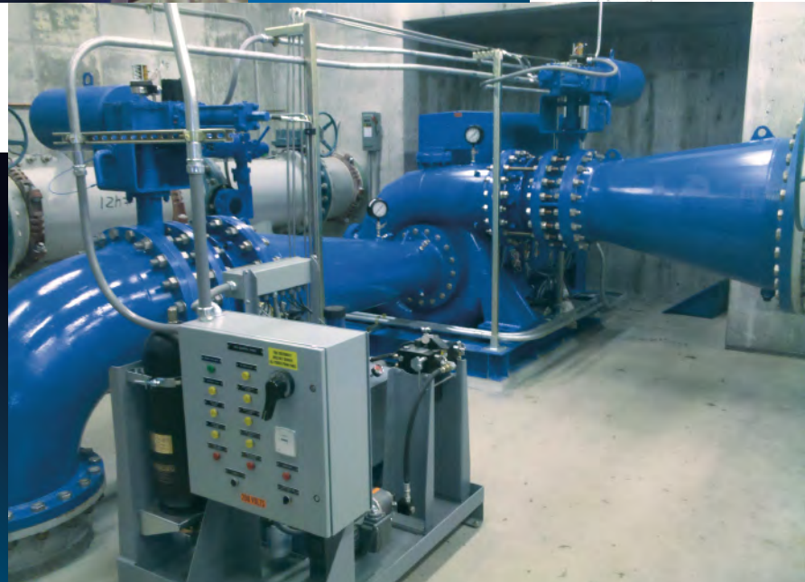
Part of a conduit system, this Canyon Hydro Francis-type turbine sits inline with a water supply pipeline for the City of Logan, Utah.
