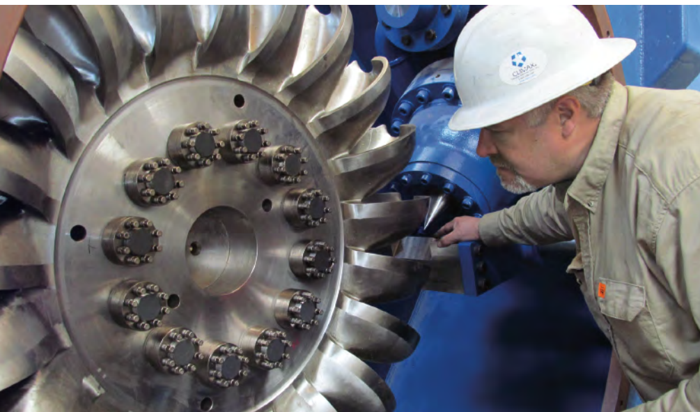
Canyon owner Richard New inspects the runner mounting bolts during installation of a 5MW Pelton system.
