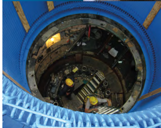
After inspection showed significant wear, Canyon built new runner buckets, deflectors and nozzle components for this 25MW Pelton system.
