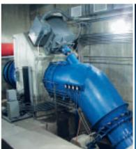
Located near Logan, Utah, this 300 kW Canyon Hydro system utilizes a Kaplantype turbine operating under 9 meters (30 feet) net head, with a design flow of 4.05 cubic meters per second (143 cfs).
