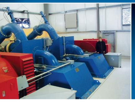
Located in British Columbia, Canada, this Canyon Hydro system uses twin Pelton turbines producing 3,000 kW each, from 316.8 meters (1,040 feet) net head. With technician Spencer New.
