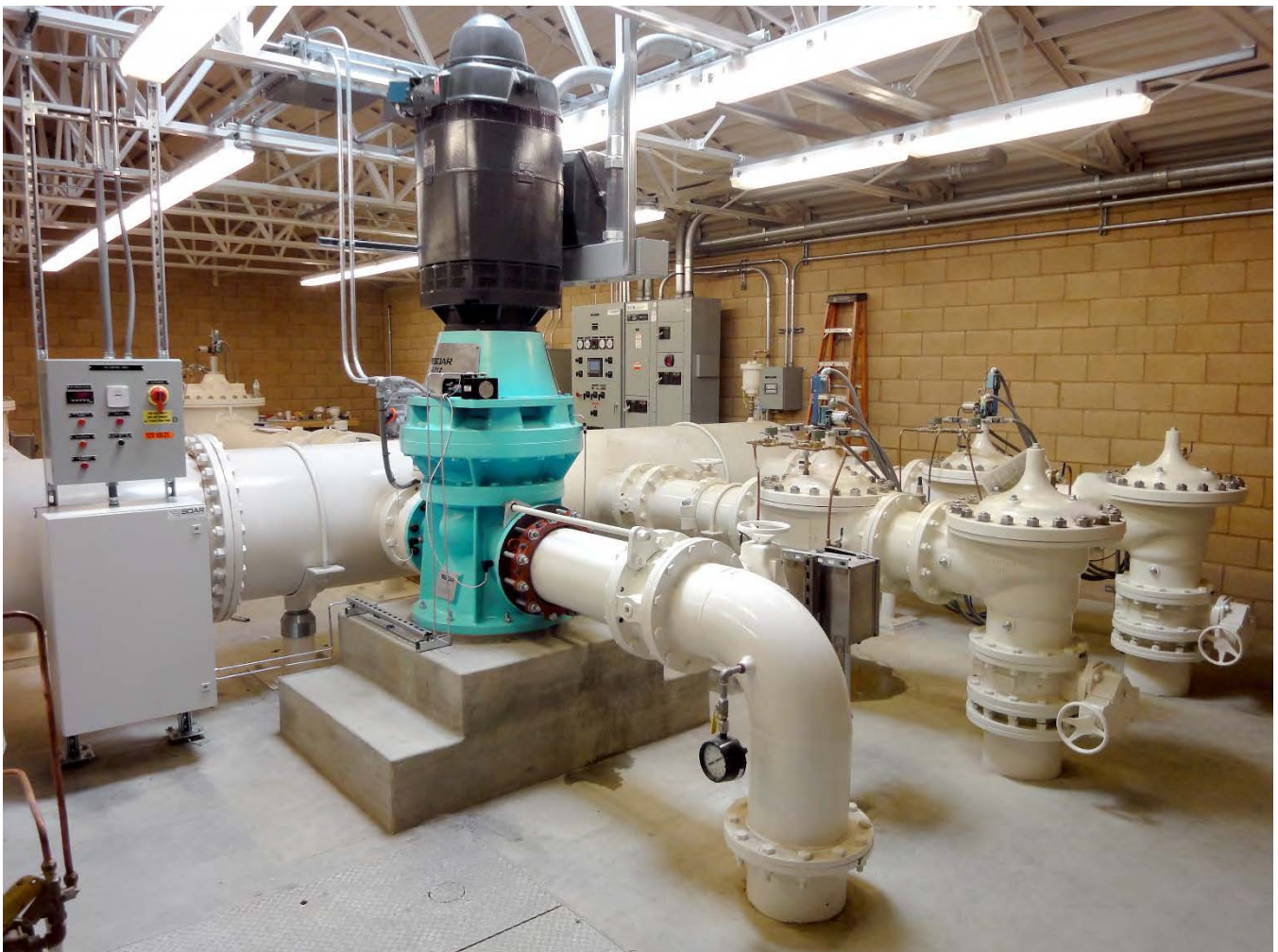
Canyon Hydro ILT-12 Turbine Installation
