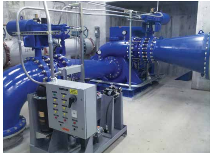
The City of Logan, Utah installed a Francis turbine to replace a pressure reducing valve
