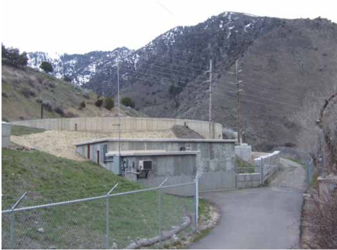
The pressure control vault houses the turbine and bypass PRV
