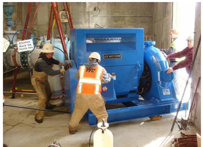
The City of Logan, Utah installed a Francis turbine to replace a pressure reducing valve
